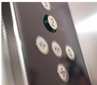
Elevator and transport systems
